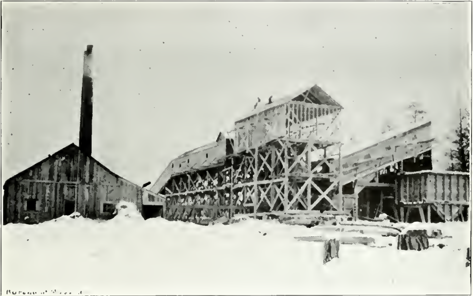
Princeton Colliery—Headworks and Tipple.
